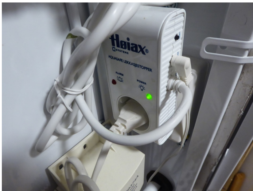
Styringsenhet – her i normal drift, Power lampe lyser
